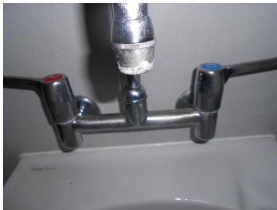
Picture 6: Lime-scale on nozzle of tap
